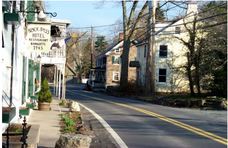
Village of Lumberville, Solebury Township
