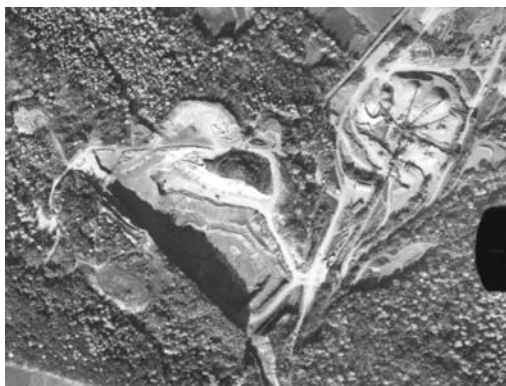
Aerial photograph of the J. T. Dyer diabase aggregate quarry, Berks County, in 1979.
