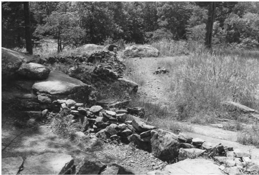
Figure 4-9. Stone breastworks on slope of Little Round Top between Sites G and H . How much of this stonework is original is debatable, but the walls are apparently in their original positions as built by men of the 44 th and 140 th New York on the night of July 2/3 (Adelman, 2000).
